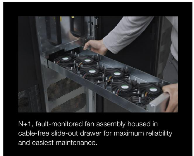
N+1, fault-monitored fan assembly housed in cable-free slide-out drawer for maximum reliability and easiest maintenance.
